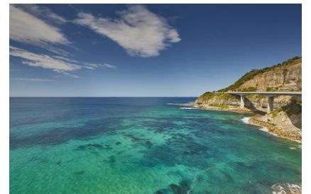
Sea Cliff Bridge, Clifton
